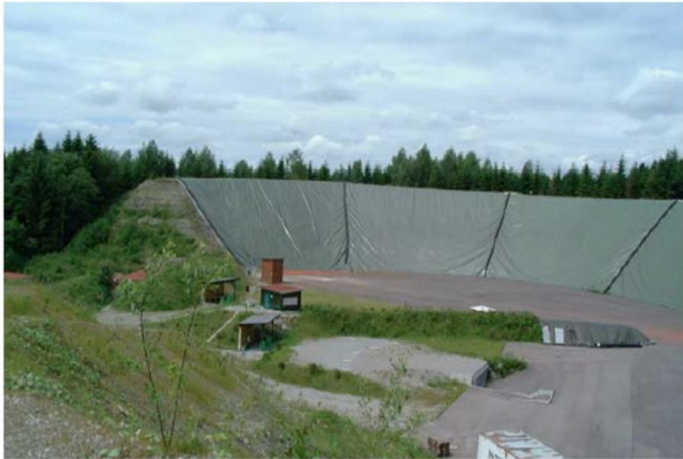
Figure A.5 Example of a range with a horizontal and a vertical barrier (Bavarian StMLU, 2003)
