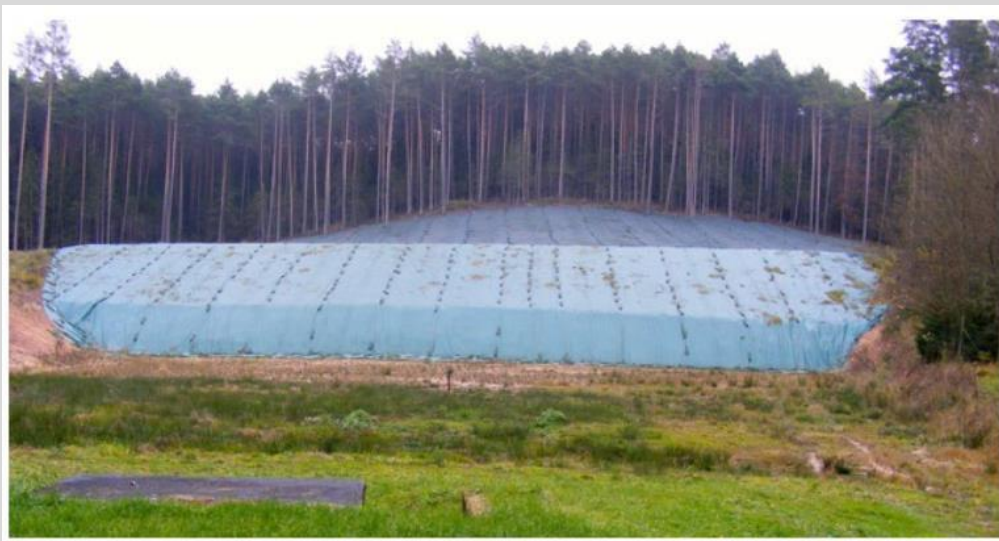
Figure A.4 Example of a horizontal barrier (Bavarian LFU, 2014)
