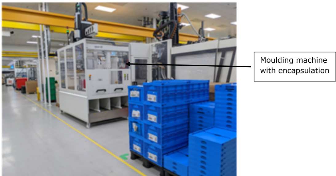
Figure 9-5 Moulding machine encapsulated with local exhaust
