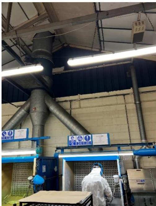
Figure VIII-1: Open spray booth where exhaust air from three booths is emitted via one stack
