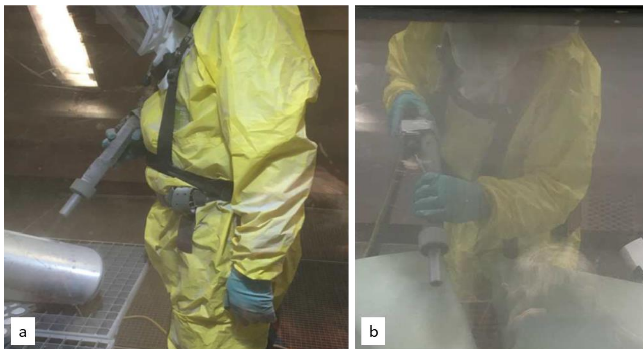
Figure 9-9: Worker performing media blasting in a room/hall (a + b)
