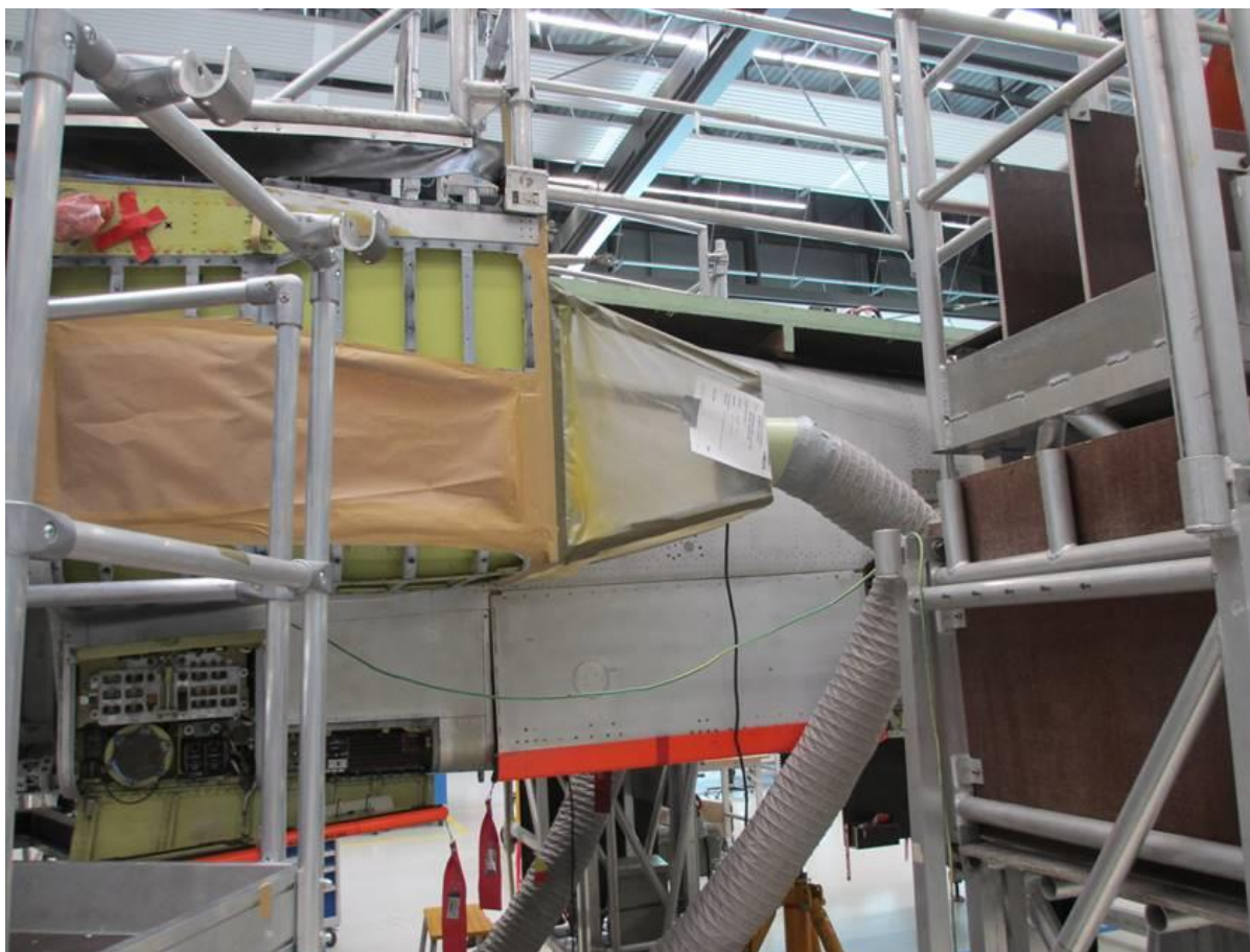
Figure 9-2: Example for a “tent” with mobile LEV installed in a working hall to perform spraying outside of a spray room/booth/hangar directly on the aircraft
