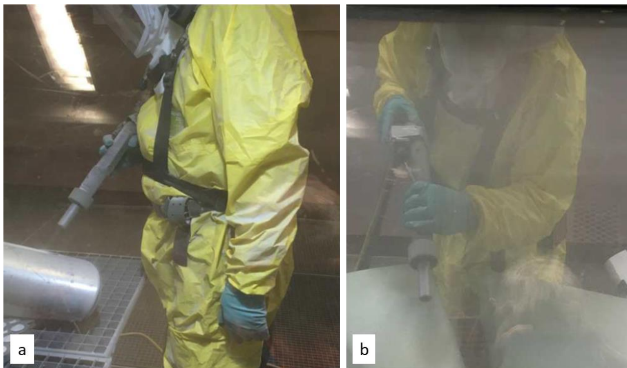
Figure 9-9: Worker performing media blasting in a room/hall (a + b)
