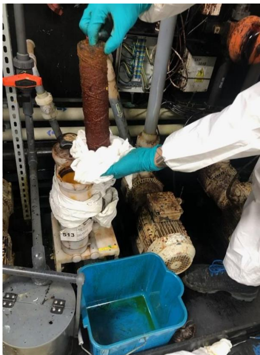
Figure 9-13: Maintenance of equipment - Filter change
