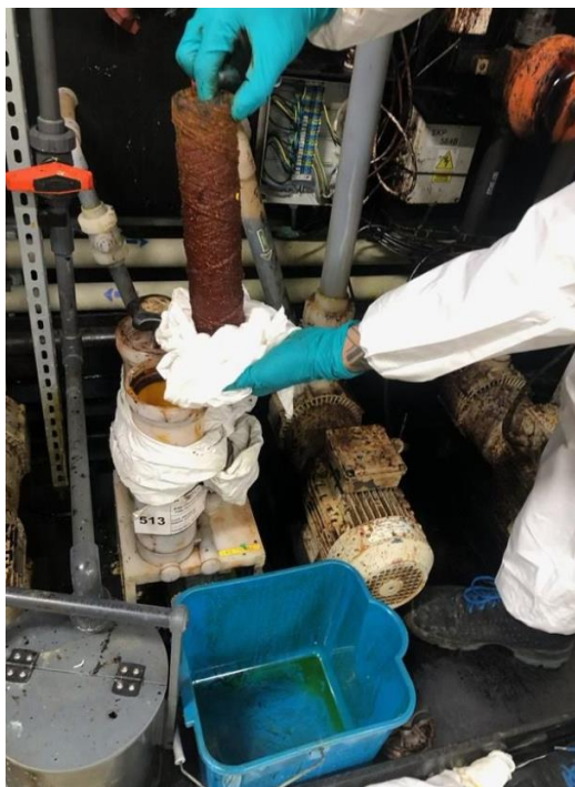
Figure 9-13: Maintenance of equipment - Filter change
