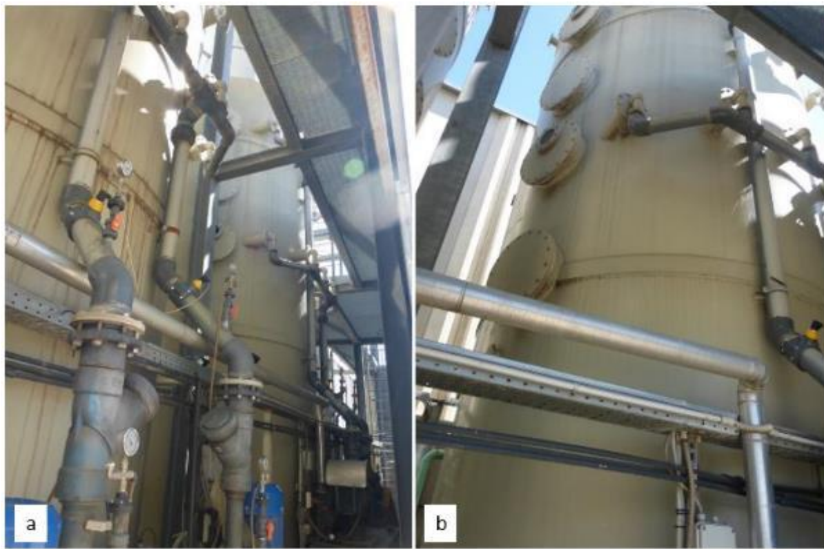
Figure 9-4: Wet scrubber (a + b)
