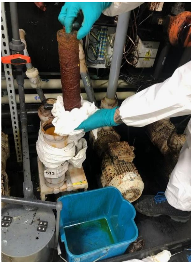
Figure 9-13: Maintenance of equipment - Filter change
