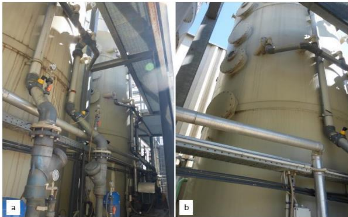
Figure 9-3: Wet scrubber (a + b)
