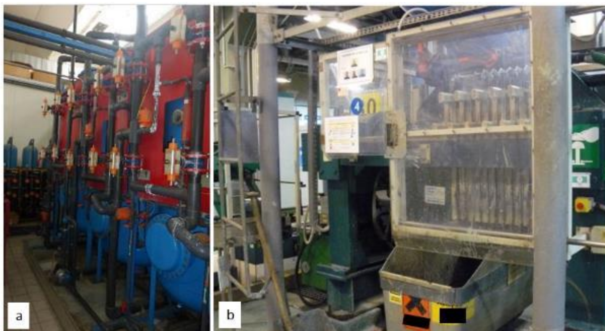
Figure 9-4: Water deionisation tanks for wastewater treatment (a) and filter press for separation of the filter cake (b)
