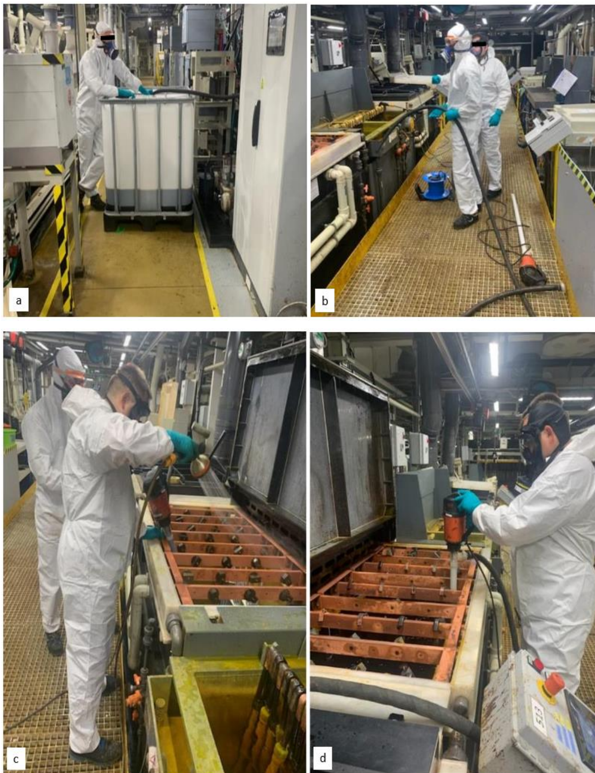
Figure 9-13: Bath emptying by transfer of old bath solution into an IBC (a) and bath cleaning with a hose and wet and dry vacuum cleaner (b, c, d)
