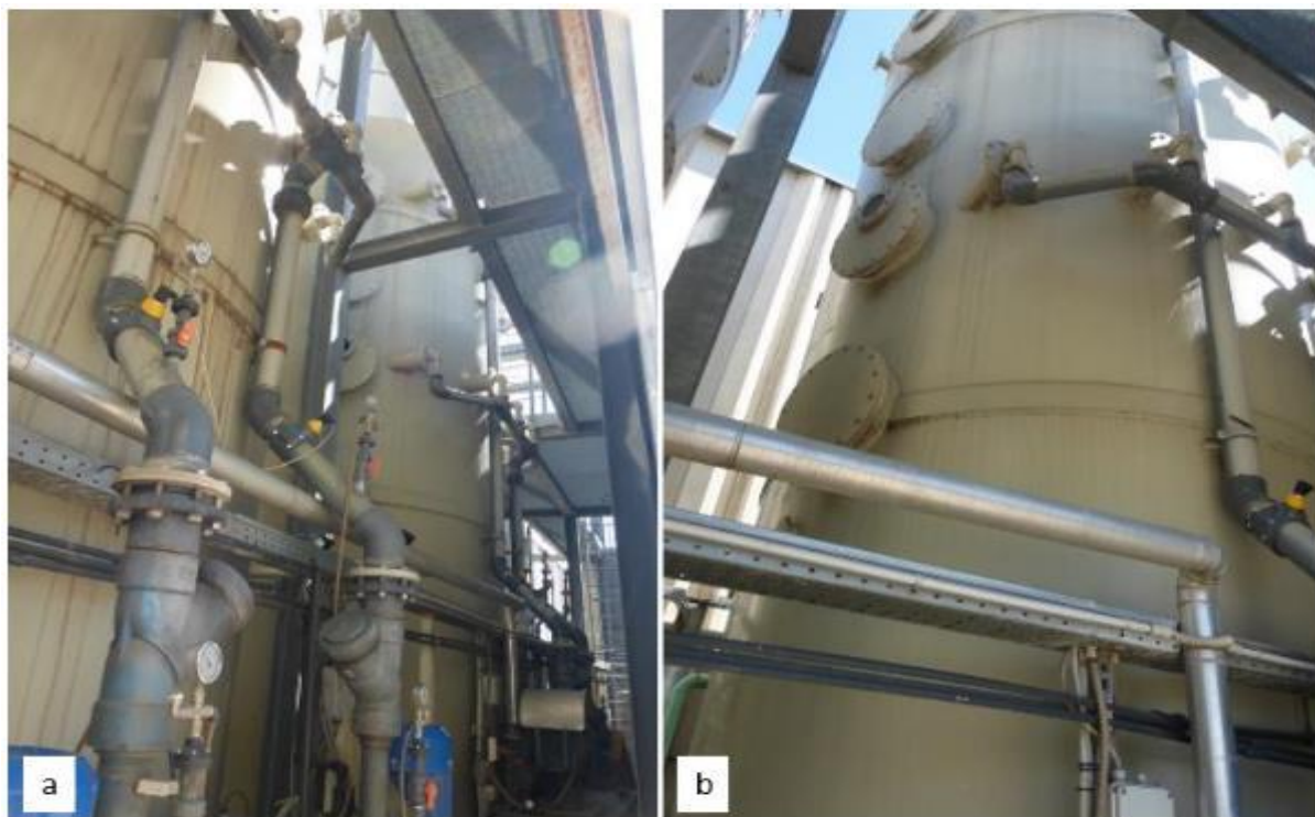
Figure 9-4: Wet scrubber (a + b)
