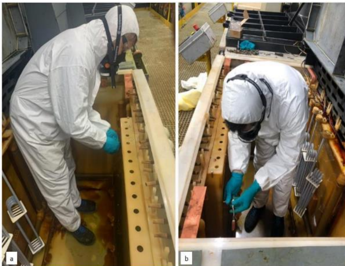
Figure 9-15: Cleaning of equipment (a + b)
