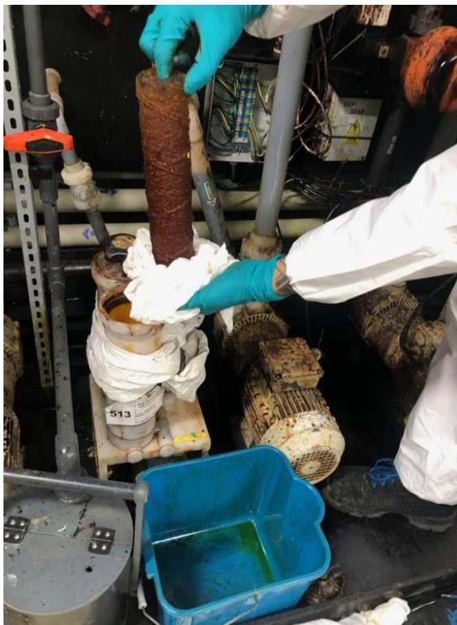
Figure 9-14: Maintenance of equipment – Filter change
