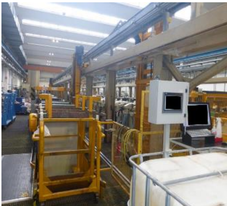
Figure 9-6: Automatic line with control area in front of automatic line (at the monitor)
