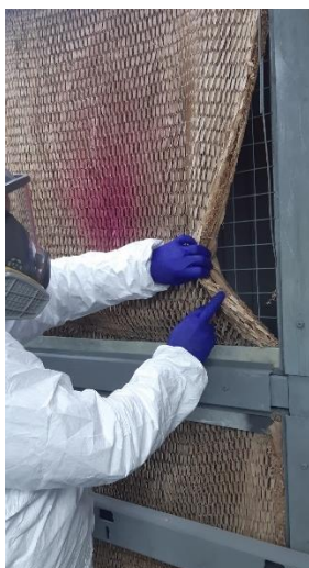
Figure 9-10: Changing of filters in spray booth
