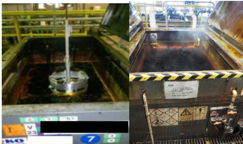
Figure 9-2: Treatment bath for pre-treatment (a + b)
