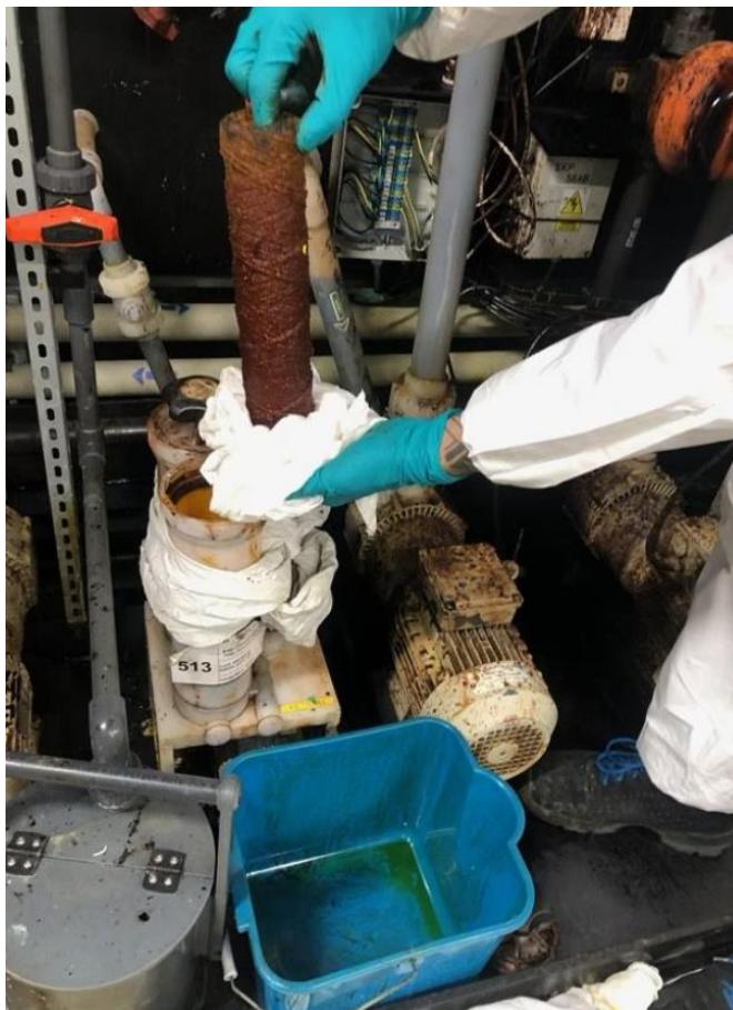
Figure 9-13: Maintenance of equipment - Filter change
