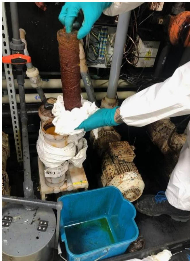
Figure 9-14: Maintenance of equipment - Filter change
