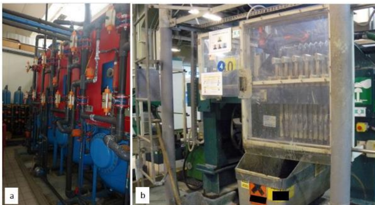
Figure 9-5: Water deionisation tanks for wastewater treatment (a) and filter press for separation of the filter cake (b)
