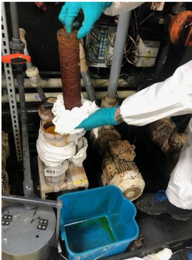
**Figure 9-11: Maintenance of equipment - Filter change**
