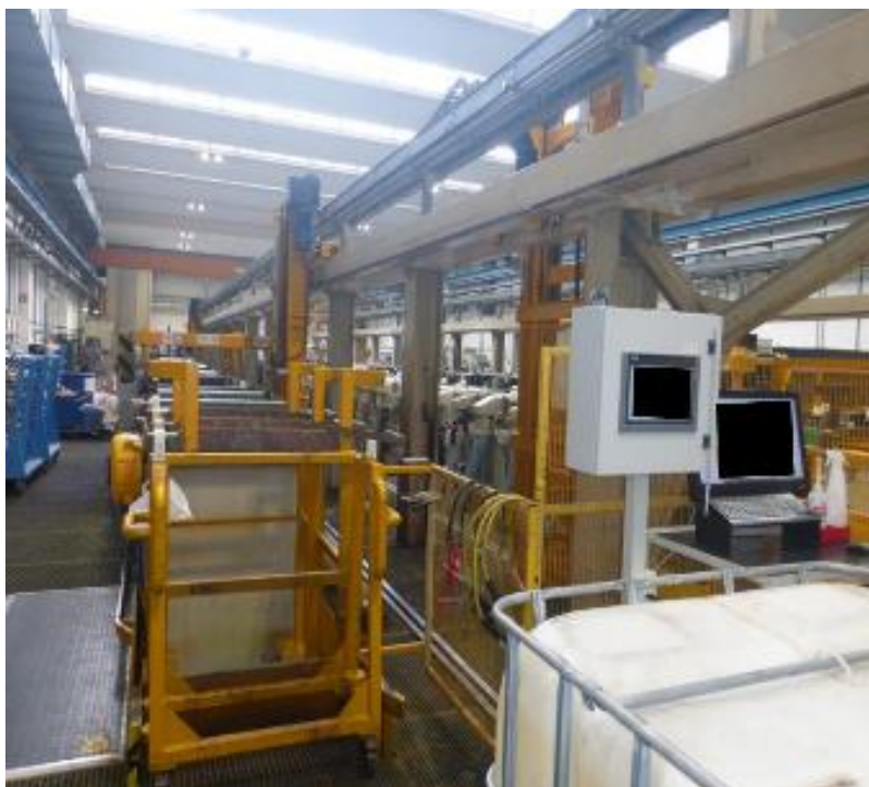
Figure 9-7: Automatic line with control area in front of automatic line (at the monitor)
