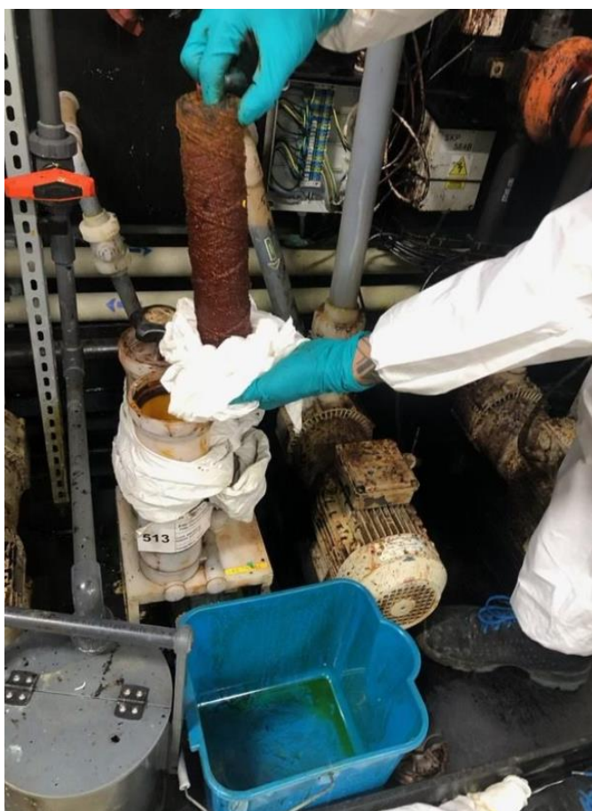
Figure 9-15: Maintenance of equipment - Filter change
