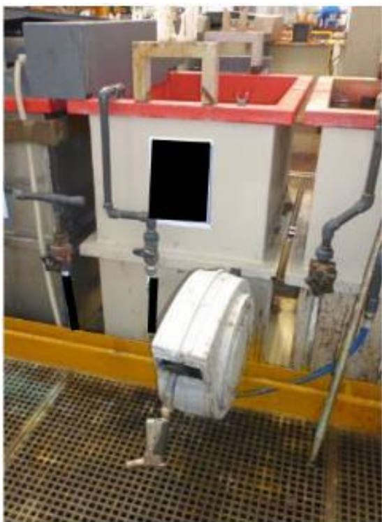
Figure 9-9: Hose for cleaning the edges of the tanks and the walkways surrounding the baths
