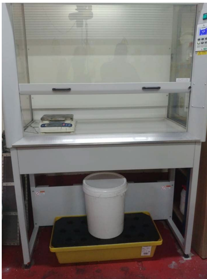
Figure 18: Photograph of new fumehood installed in chemical storeroom
