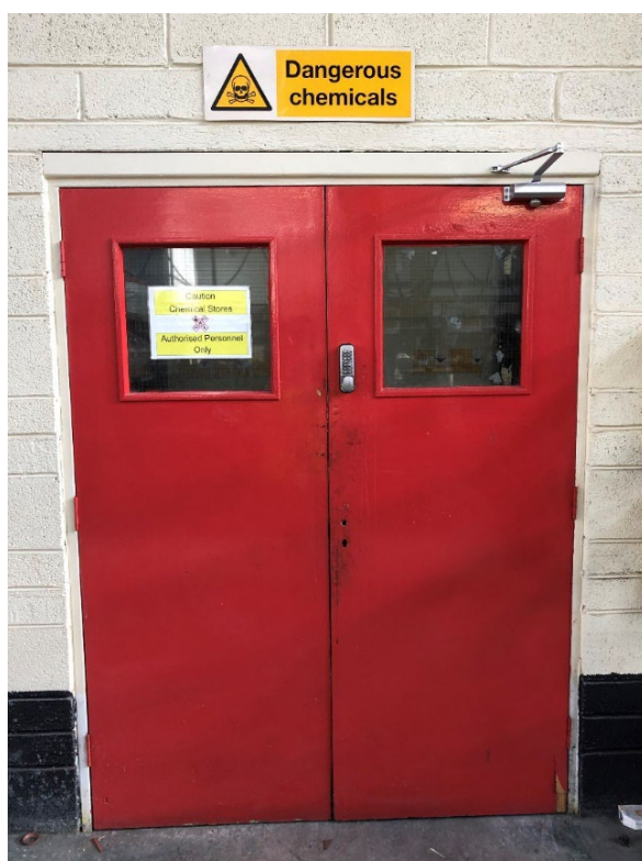
Figure 6: Photograph of keypad-locked door to chemical stores
