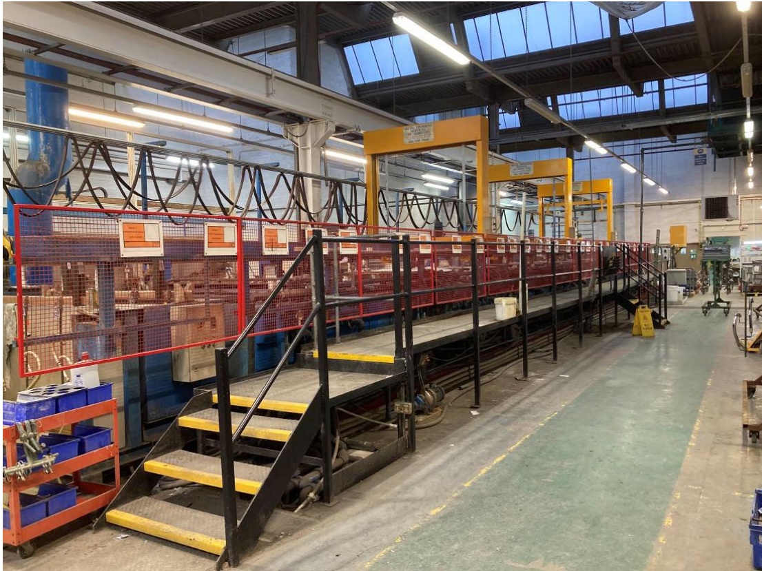
Figure 19: Photograph of plating line walkway
