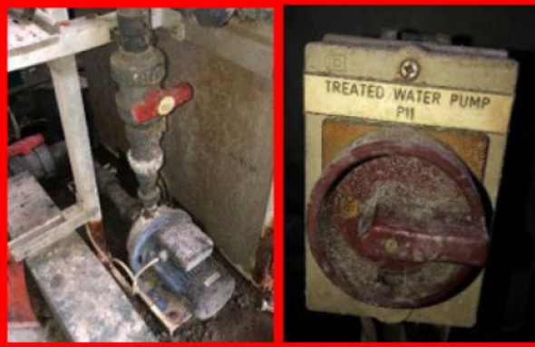
Valve closed & Pump Off
