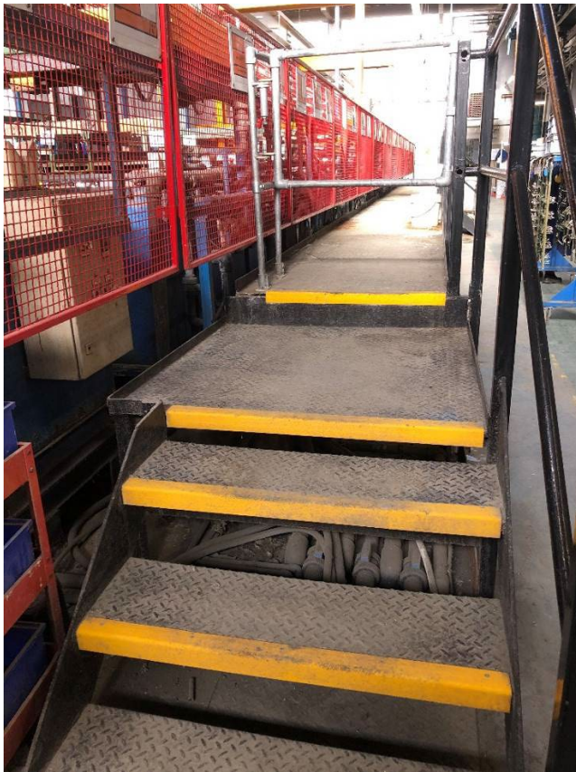
Figure 20: Photograph of gated walkway on plating line
