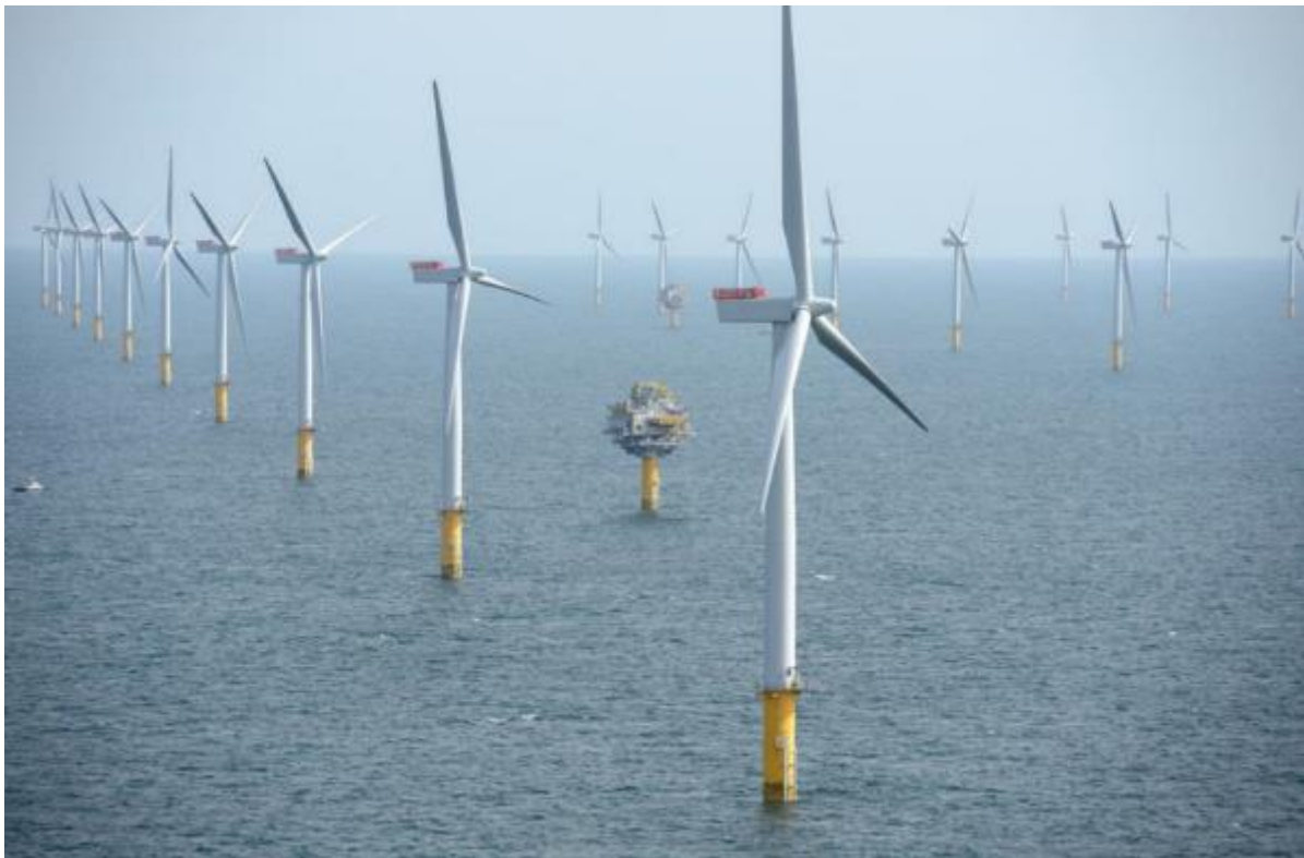
Figure 9. Offshore wind park showing wind turbines as well as a substation used to connect the turbines to the power grid
