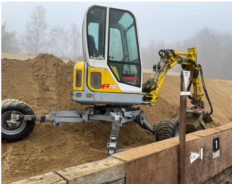
Figure 4 Mechanical recovery of lead in a sand stop butt at the National Shooting Centre, Bisley (photograph taken 14/2/23)
