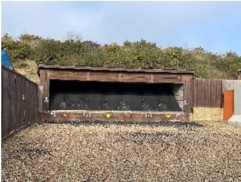
Figure 3 Rubber granule stop butt for a range at the National Shooting Centre, Bisley (photograph taken 14/2/23)
