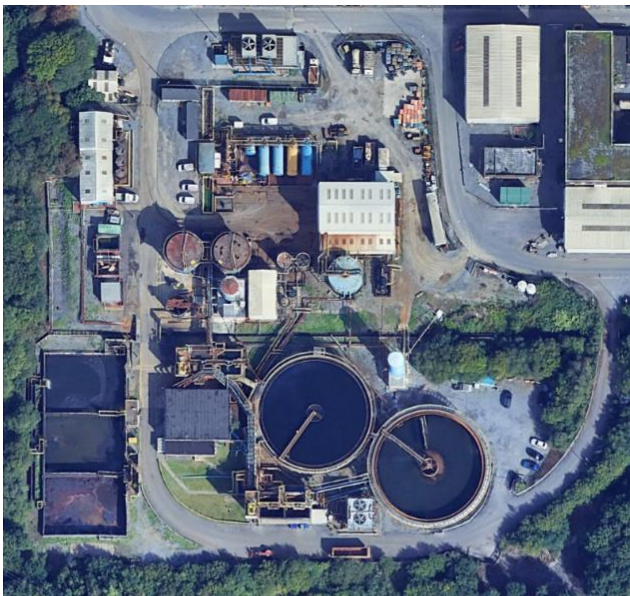
Figure 9: Wastewater treatment plant
