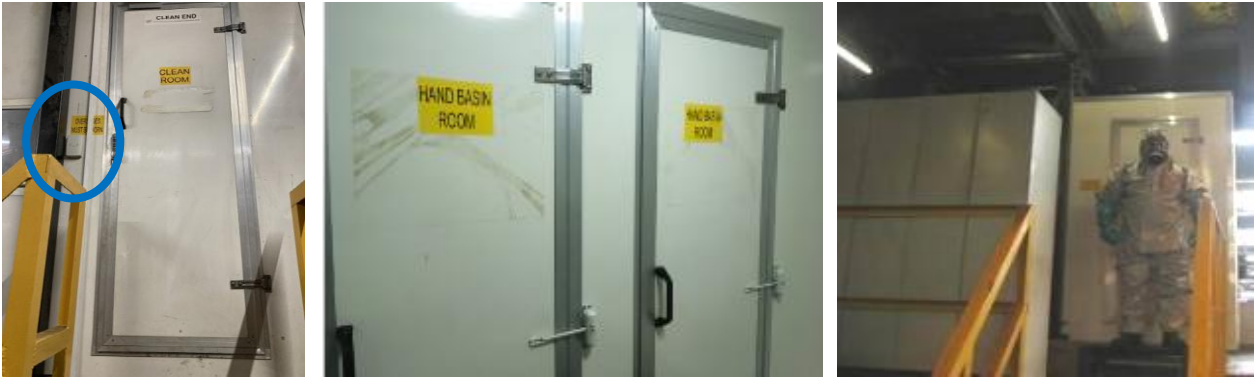
Figure 21: Left: Access to the decontamination block with magnetic lock highlighted. Centre: Two closed room to dress and disrobe PPE. Right: Fully dressed operator leaving the decontamination block.
