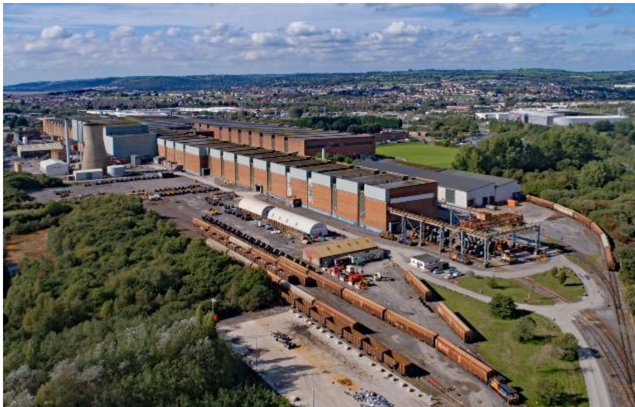
Figure 1: The Trostre Works in Llanelli, Carmarthenshire
