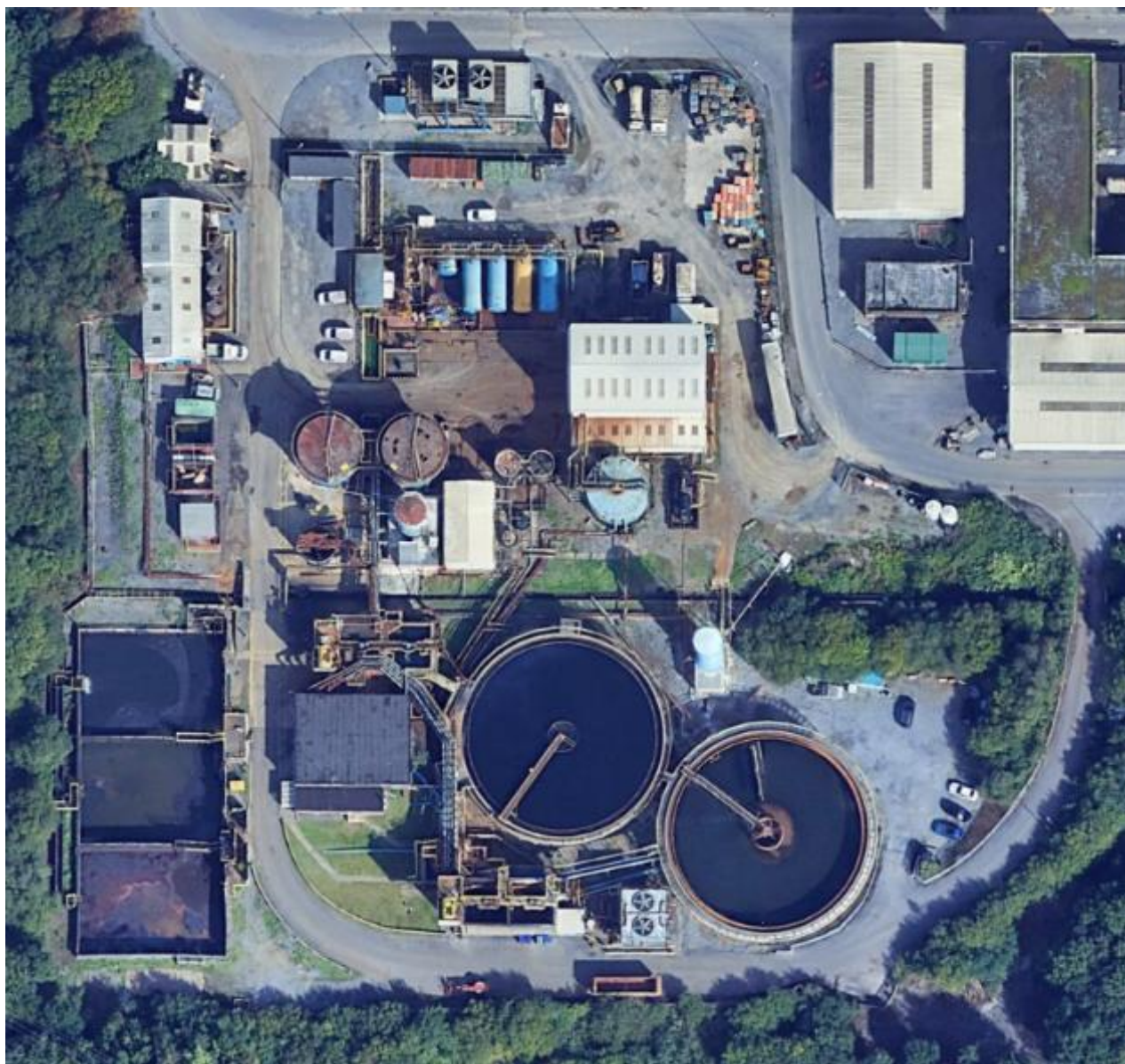
Figure 8: Wastewater treatment plant
