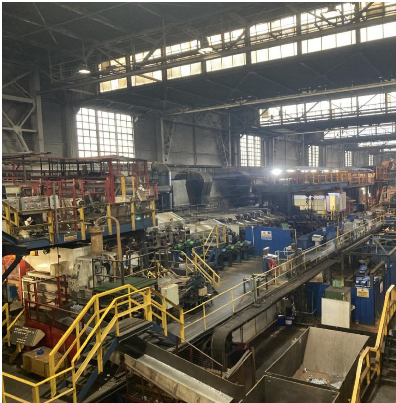
Figure 5: Electrolytic chromium coating line no. 4 (ECCS4) within Area 3 of the Trostre Works
