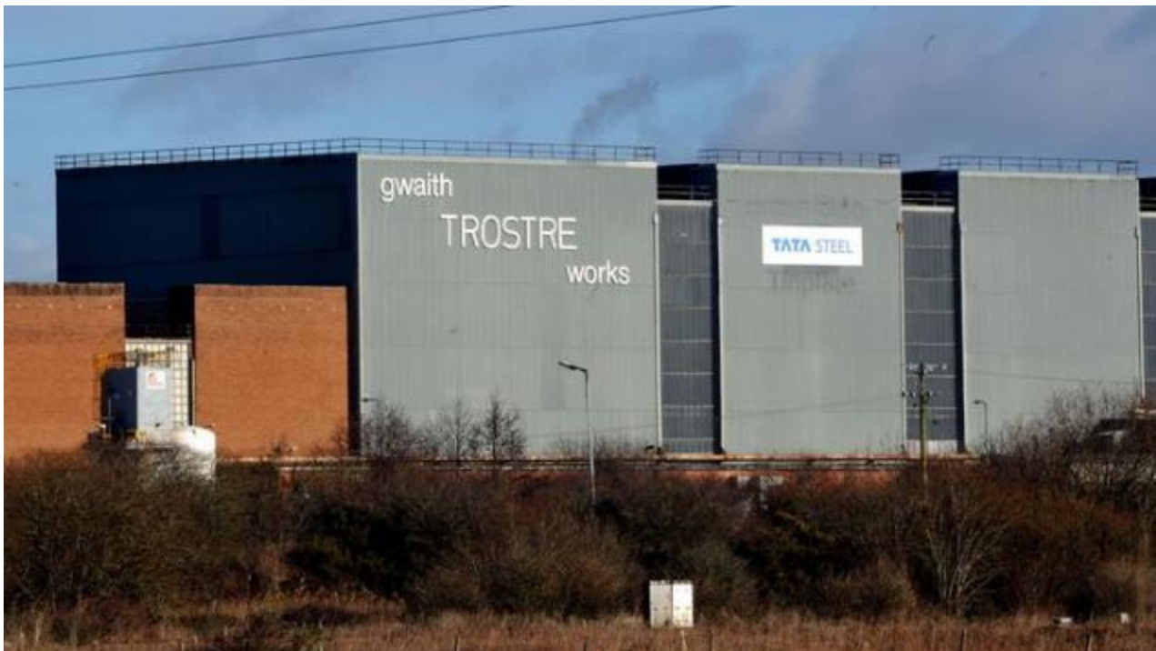
Figure 1: The Trostre Works in Llanelli, Carmarthenshire
