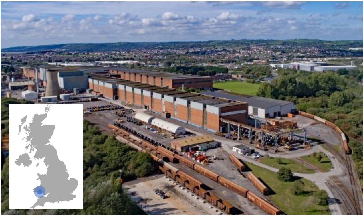
Figure 4: The Trostre Works in Llanelli, Carmarthenshire
